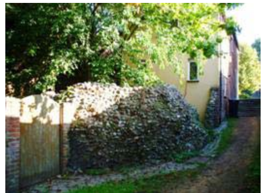
Oak Street steps to the river and the remains of a City Wall tower
