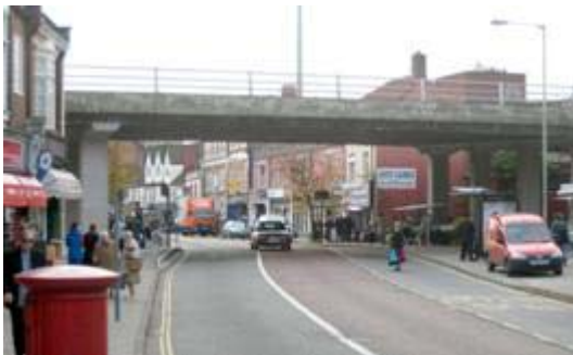
Magdalen Street flyover
