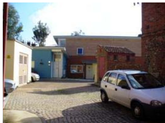
modern development to the rear of Zipfel House, Magdalen Street
