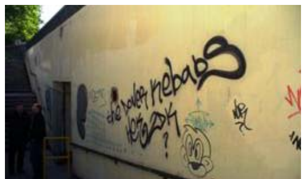
St Crispin's underpass
